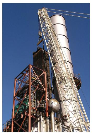
After operating for 10 years, a cogeneration plant with a single Nooter/Eriksen HRSG servicing a refinery had begun experiencing multiple tube leaks in their HP Economizer Coils. The cause of the leaks was determined to be underdeposit corrosion due to iron deposits. The feedwater quality could not be addressed directly as it is supplied by the refinery and is beyond the control of the HRSG operators.
